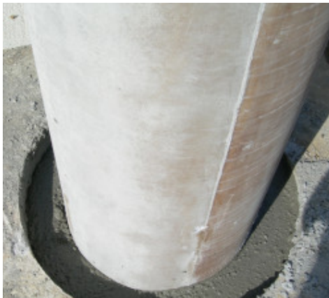
Anchoring of precast pillar
