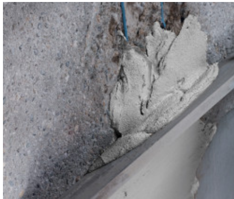
Smoothing of Planitop Smooth & Repair Zero with a straight edge
