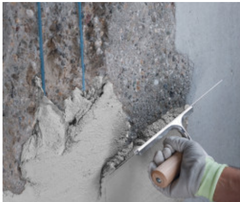
Application of Planitop Smooth & Repair Zero with a spatula
