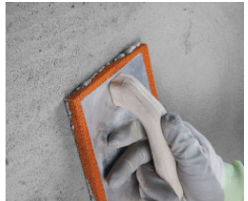
Tamping Planitop Smooth & Repair Zero
